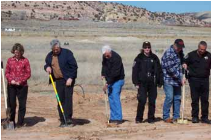
L to R: Lisa Nielsen of UBAOG, Commissioner Collett, Mayor Dickison, Christy Kendrick, Commissioner Leith and Lt. Rick Harrison dig in to officially break ground for the county's new affordable housing.
